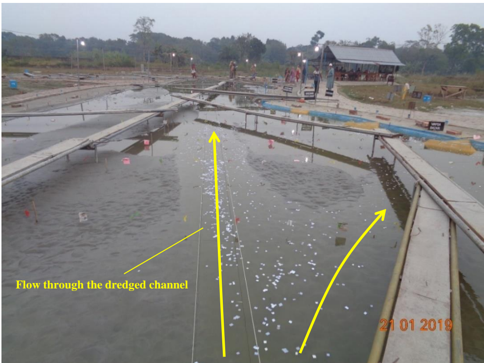
Fig. 4. Flow through the dredged channel at low flow (T6)
