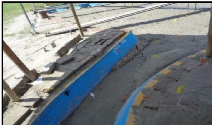
Fig 7. Launching apron at the off-take mouth along the right bank
